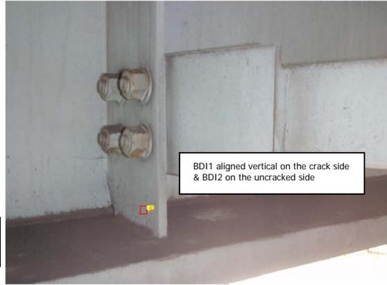
Figure 5. No Sign of Cracking at G3B3D3 (Girder 3 Bay 3 Diaphragm 3) and one
