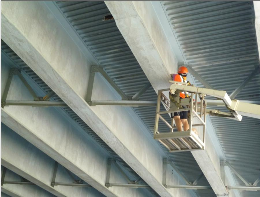
(a) Installing piezo film AE sensors on connection plate
