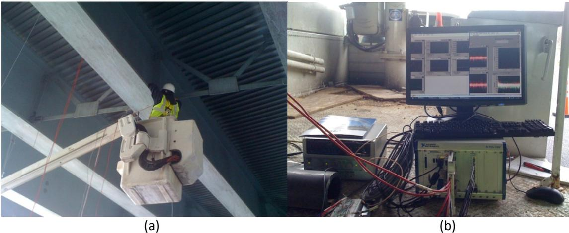
Figure 10. (a) Installing AE sensors and wiring; (b) AE data acquisition
